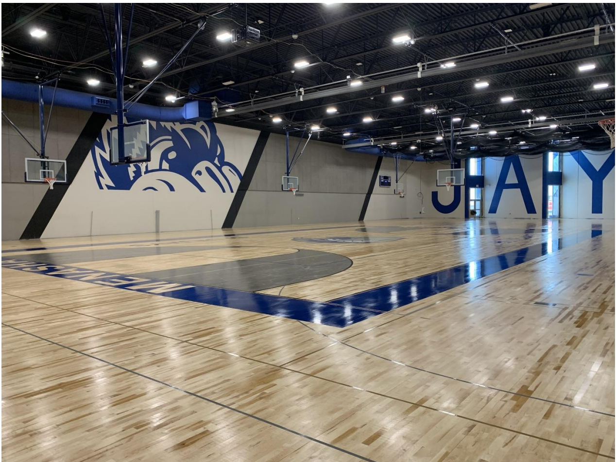
26. Area 6 - Gym floor appears to be installed, striped, painted, and sealed.
